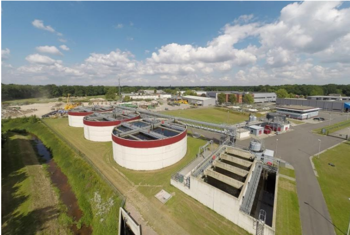
Figure 21. Epe waste water treatment plant was the first municipal waste water treatment plant with a full Nereda process, commissioned in May 2012.
