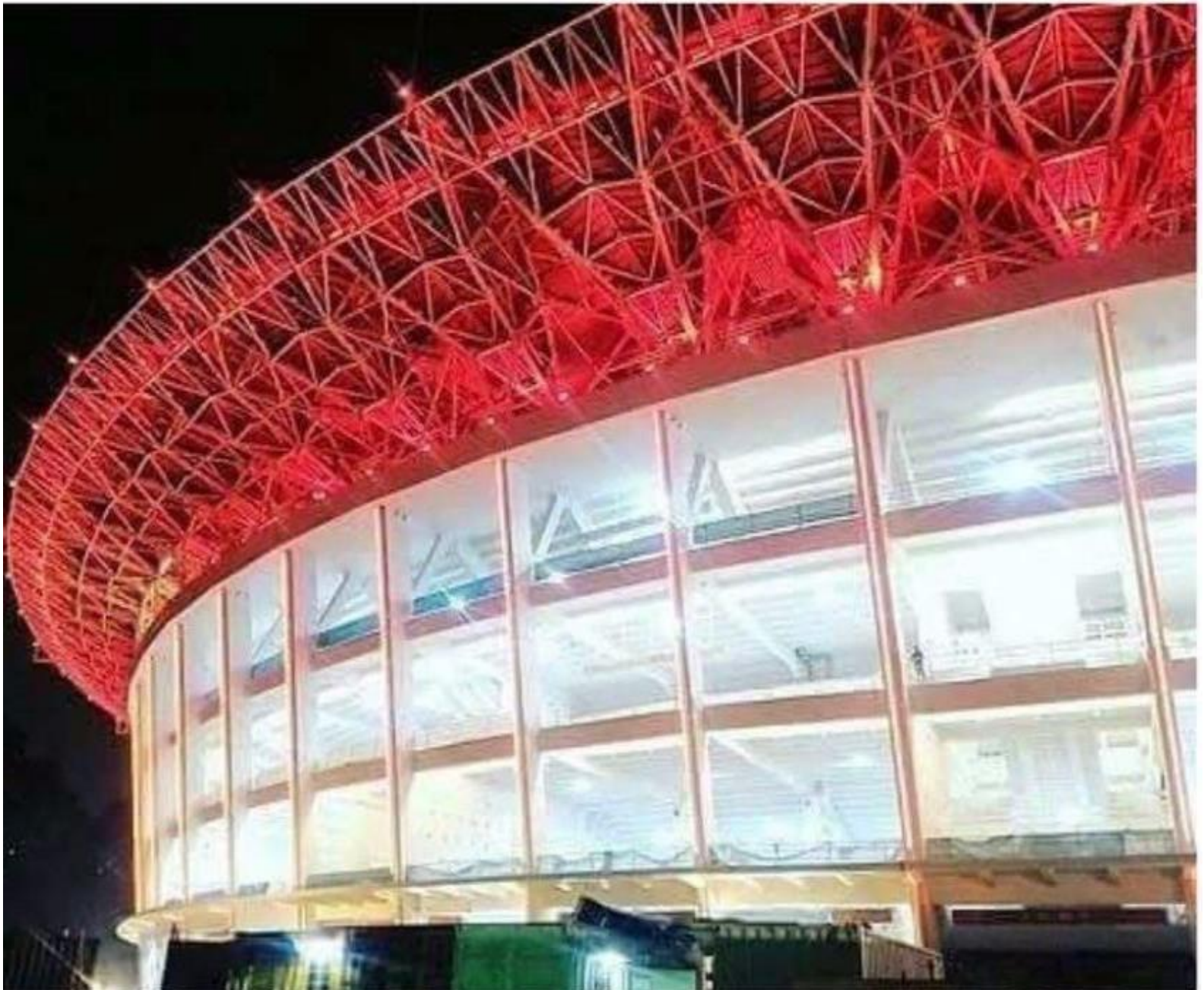
Figure 45. The New of Gelora Bung Karno Main Stadium around 2018s and Renovation under PT Adhi Karya, Tbk (Source: PT Adhi Karya, 2018)
