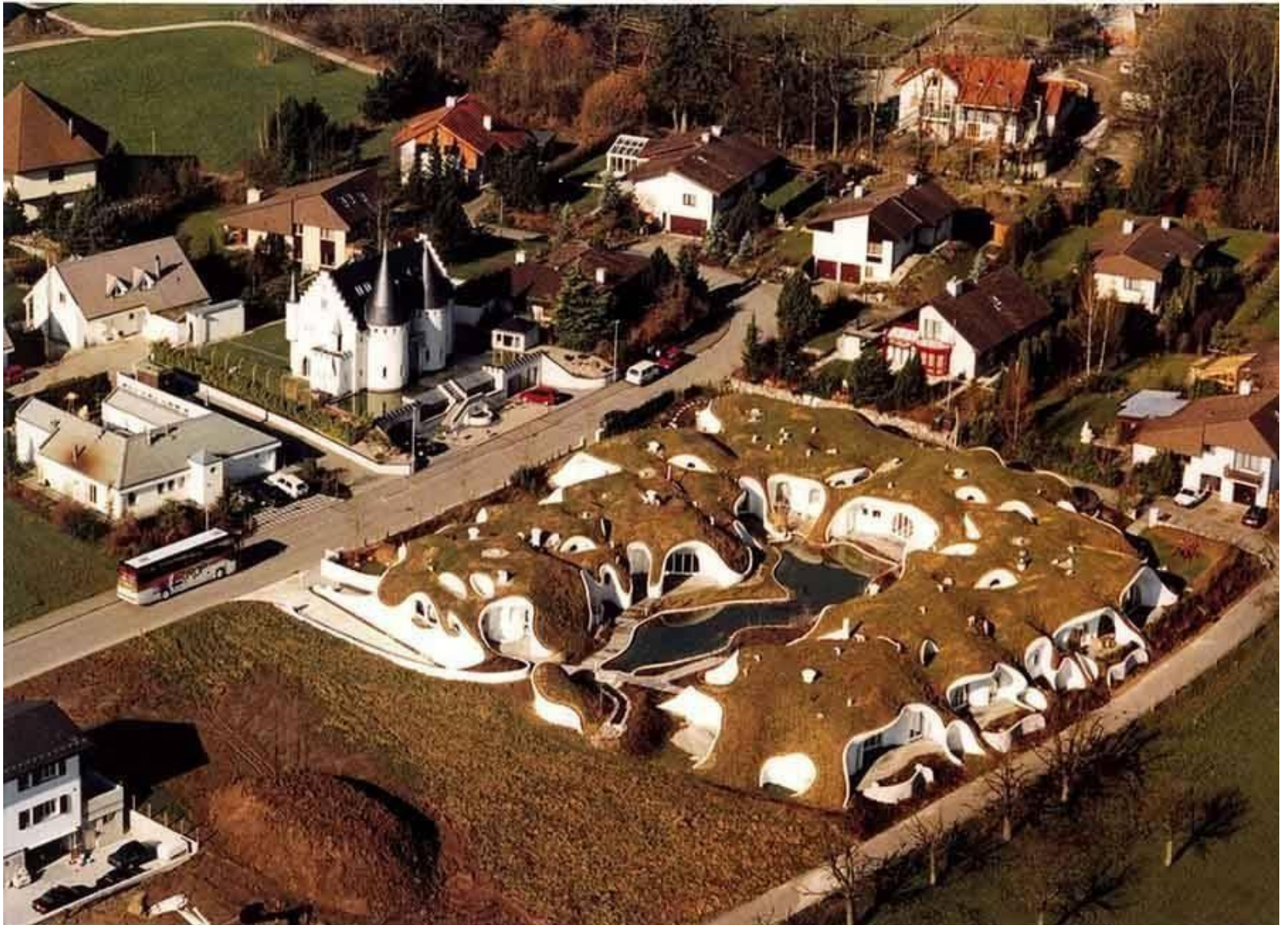
Figure 3. Earth Houses of Switzerland Source: harpersbazaar.co.id
