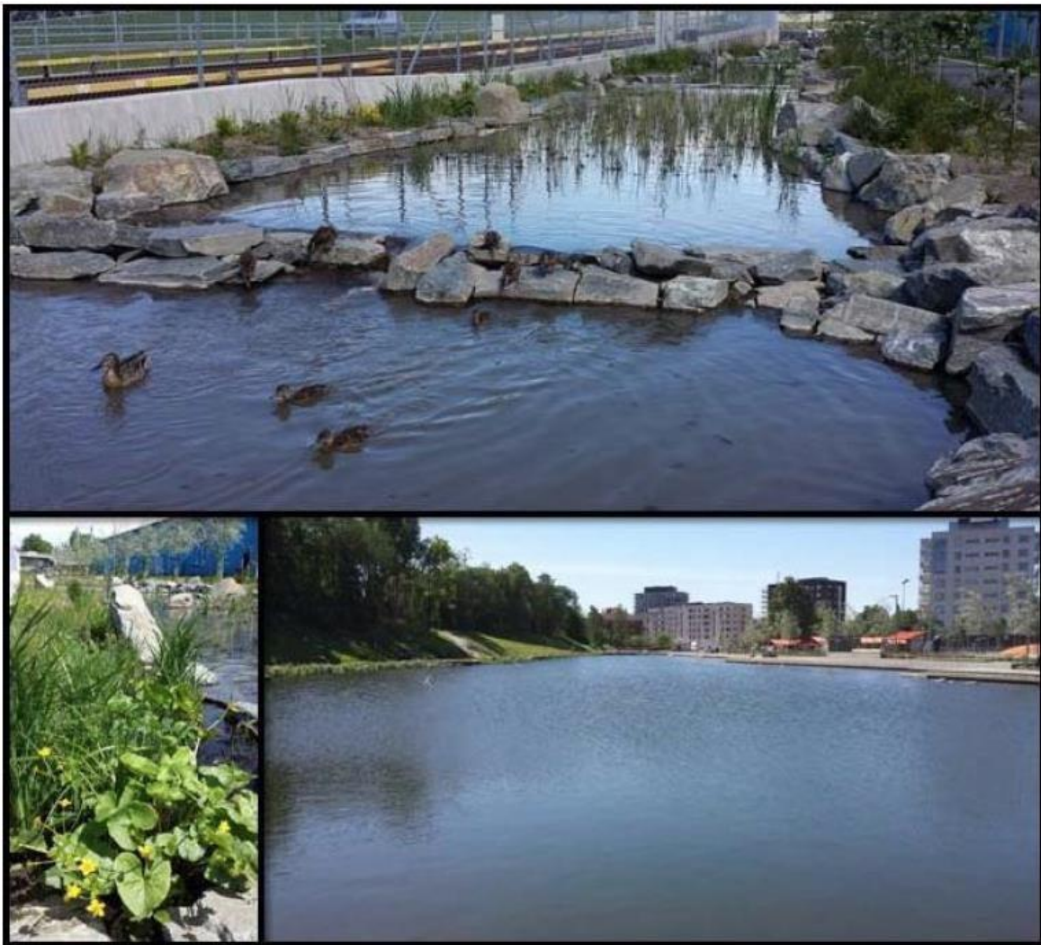
Figure 24. Teglverksdammen is a large scale reopening of the stream Hovinbekken. All together 650 meters of the stream has been opened, with sedimentation basins, water rapids, indigenous plant species, a small lake, shallow waters, with dense vegetations.
