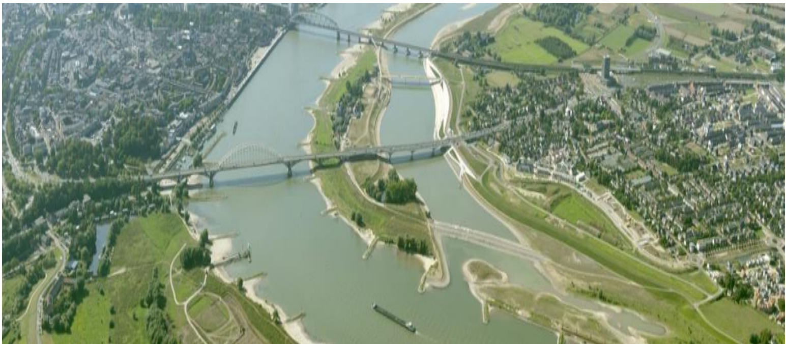
Figure 35. Waal river and its secondary channel with surrounding land uses in Nijmegen City and Lent Town, The Netherlands.
