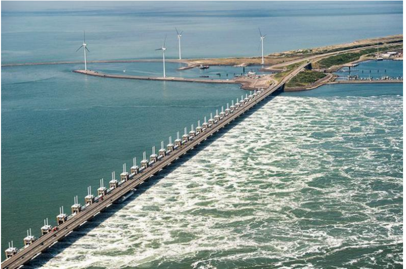
Figure 34. The Oosterscheldekering (Eastern Scheldt storm surge barrier), between the islands Schouwen-Duiveland and Noord-Beveland, is the largest of the 13 ambitious Delta Works series of dams and storm surge barriers, designed to protect the Netherlands
